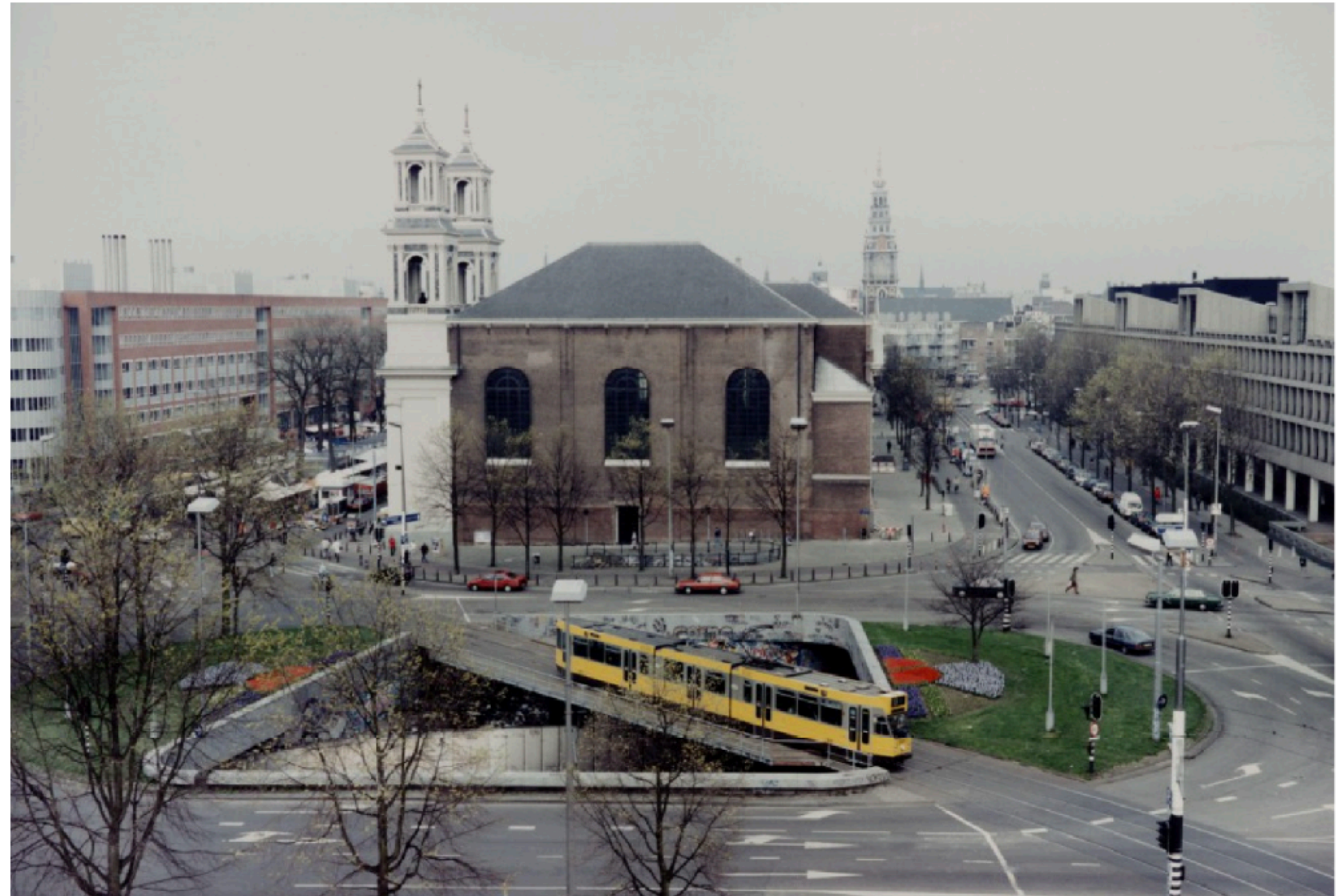
Situation around 1993: tunnels closed, no roof yet (view from the opposite side towards Waterlooplein and Zuidkerk)
